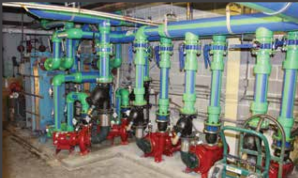
Corpus Christi Athletic Club, Corpus Christi, TX. Condenser water line retrofit.
